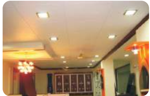
FALSE CEILING AND FLUSH JOINT
